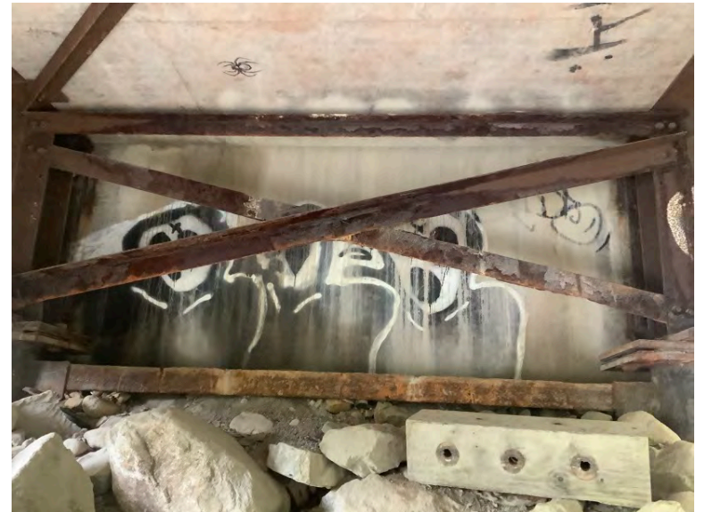
Right Bank Abutment when facing downstream
