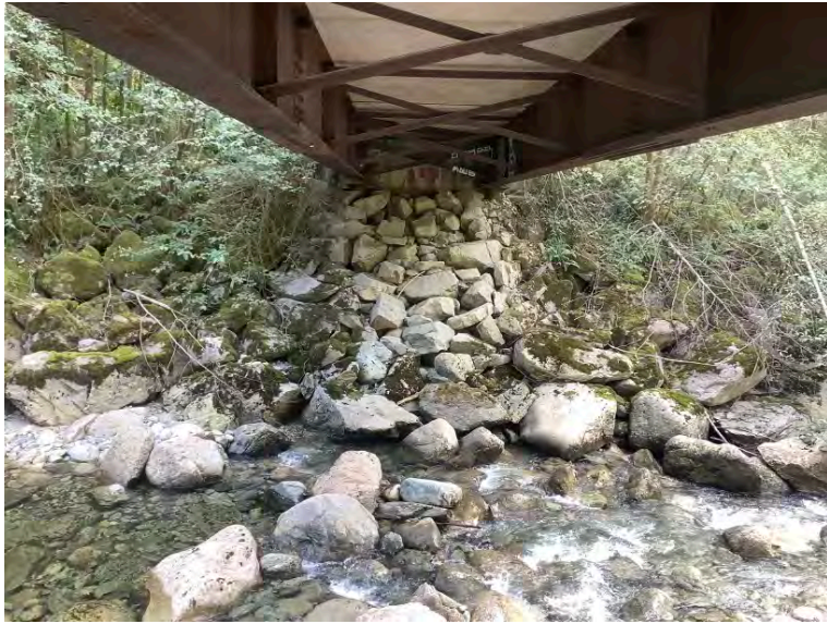
Left Bank Abutment when facing downstream
