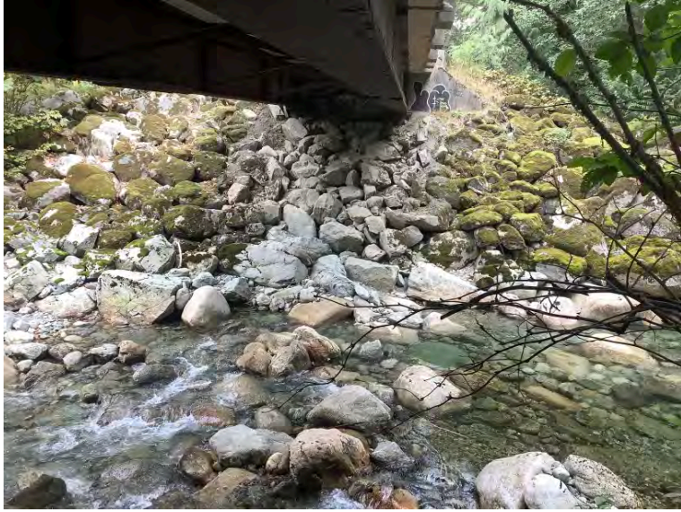
Right Bank Abutment when facing downstream
